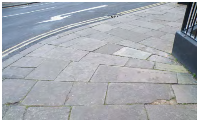
Fig 63. Stone flags at Chiswick Street, carefully cut to a radius.
