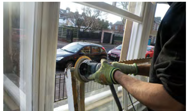
Fig 50. The refurbishment and draft stripping of a traditional sash window which if maintained will last for many decades.
