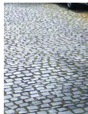
Fig 65. Dressed basalt setts at Alfred Street North and napped basalt at Hart Street are both valuable aspects of the area warranting retention and careful repair where needed.
