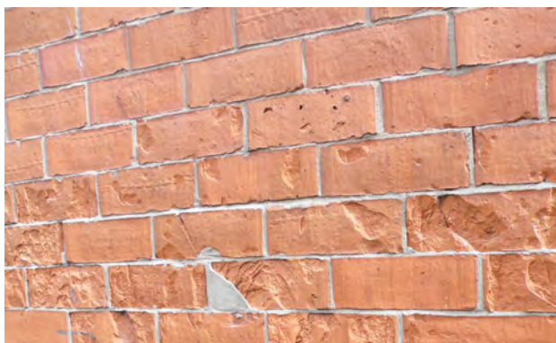
Fig 52. Spalled bricks due to the use of hard cement in repointing work instead of softer lime based mortars.
