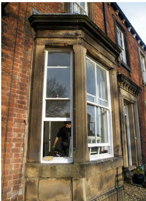
Fig 53. Vertically proportioned windows and openings are a feature of the area- this bay window is undergoing refurbishment and draft stripping to improve its energy efficiency.
