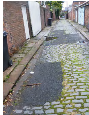
Fig 67. Loss of basalt setts to tarmac rear of Hart Street and very crude reinstatement of river cobbles to the rear of Chapel Street/Victoria Place.
