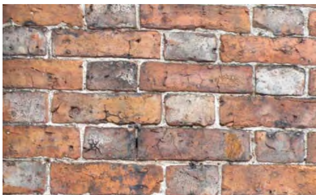
Fig 51. Distinctive chequeboard brickwork with header and stretcher bricks in contrasting colours are a feature of the Conservation Area.
