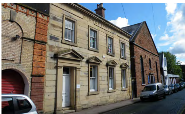
Fig 45. The Grade II Dispensary building on Chapel Street, built 1858, in sandstone ashlar with neo-classical detailing.
