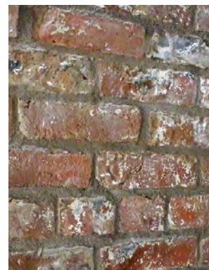
Fig 78a. Cement pointing causing spalling of bricks (left) Fig 78b. Correct pointing of bricks with lime mortar (right)
