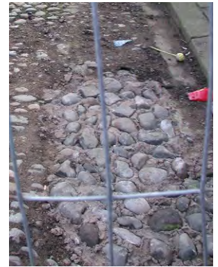
Fig 67. Loss of basalt setts to tarmac rear of Hart Street and very crude reinstatement of river cobbles to the rear of Chapel Street/Victoria Place.
