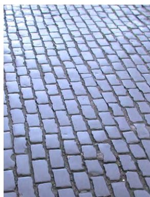
Fig 65. Dressed basalt setts at Alfred Street North and napped basalt at Hart Street are both valuable aspects of the area warranting retention and careful repair where needed.
