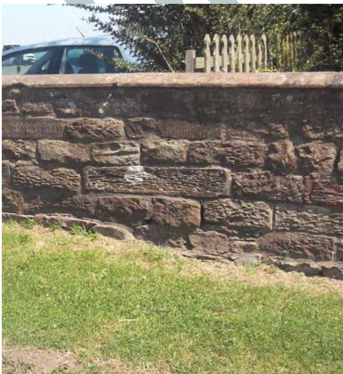
Figure 24: Reused lintols in stone boundary walls
