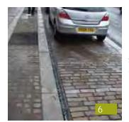
• Road markings are obtrusive, particularly in historic areas and zones of pedestrian priority. If necessary, road markings and delineation should be sensitively integrated into the paving design by a material change [6] or through metal floor studs/details [7].
