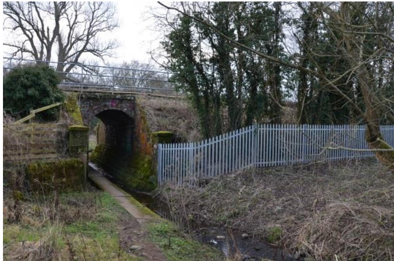
Railway bridges (LUC)
