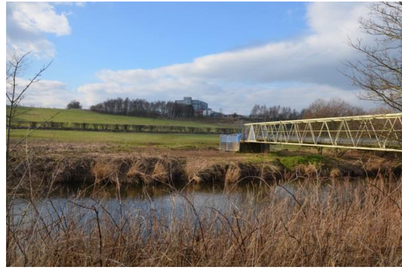
Footbridge near the print works (LUC)
