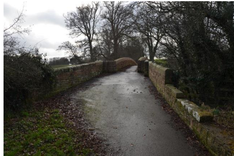
Bridge near Newbiggin Road (LUC)
