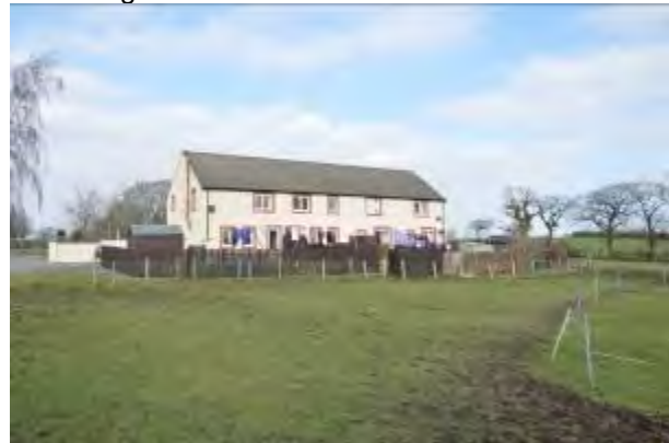
9. Smiddy Croft and land with potential for backlands development east of the village. (Also see Photo 6).
