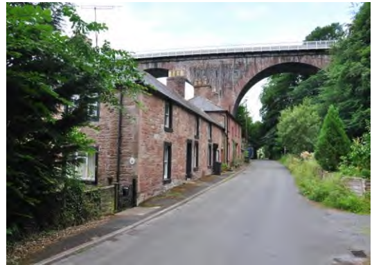
3. Impressive Corby Bridge also known as 'Wetheral Viaduct' carrying the railway track across the Eden river gorge.
