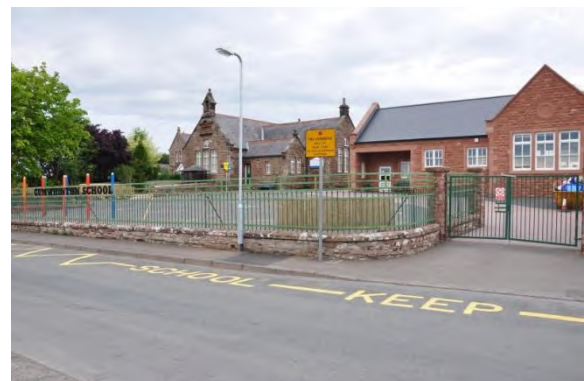
6. The attractive school has been extended in appropriate materials and adds vibrancy but feels rather detached from the village centre.
