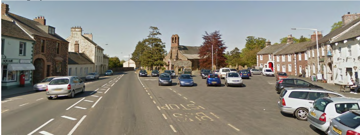
1. The Square, Dalston, (looking north) which narrows to the south and through which the B5299 passes. The Square is comprised of mainly 18 th and 19 th century buildings however some predate this, most of the buildings are listed. The red sandstone St. Michael's Church dating from the 13 th century is located at the northern end. The Square is at the centre of the wider conservation area. Many of the shops and services are located here. The Parish Council has a long standing aspiration to enhance the public realm of The Square and to make it more pedestrian friendly.
