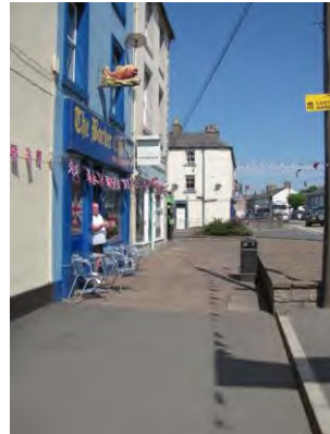
2. High Street looking south. Straight road alignment, traffic passing through the town. Wide pavements with bedding plants in low planters. Area with some 3-storey properties.
