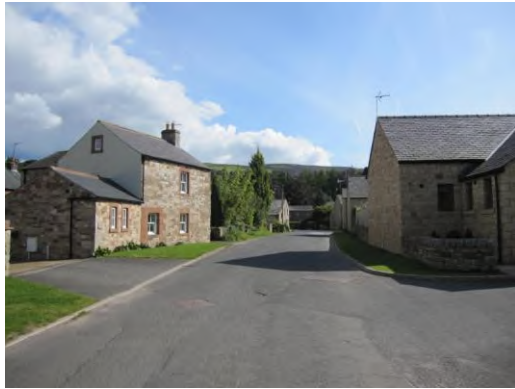
7. View south eastward towards the fells with new built housing built in sandstone.
