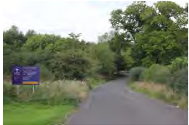
8. Looking south along the approach to the Church, which is located in a dip separated from the rest of the settlement. This is the former approach road to the village before the access was redirected over the M6.
