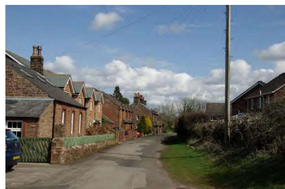
7. Railway Cottages, showing sensitive and harmonious infill next to traditional cottages backing on to Mallinson works.
