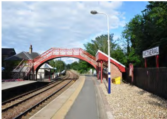
8. Wetheral Station linking this settlement to Carlisle and Newcastle via the rail network.
