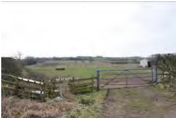
7. Wide expansive views south west from sub-station near The Oval.
