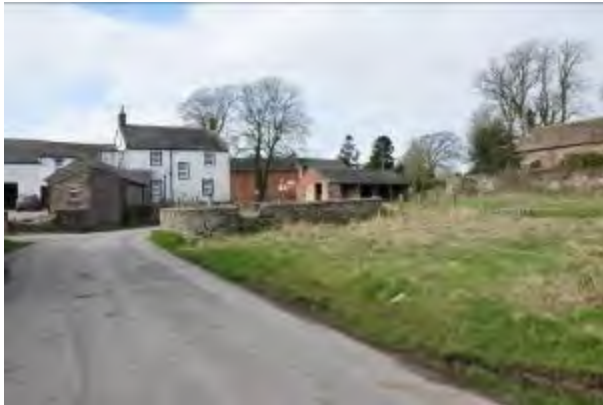
1. Approaching the junction of the north-south road through the village from the east. Back of St. Giles' Church on the right and farm house and farm buildings feature prominently in the village.
