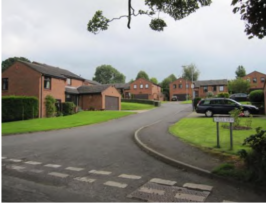
7. Castle View, building materials not in keeping with locally sourced materials
