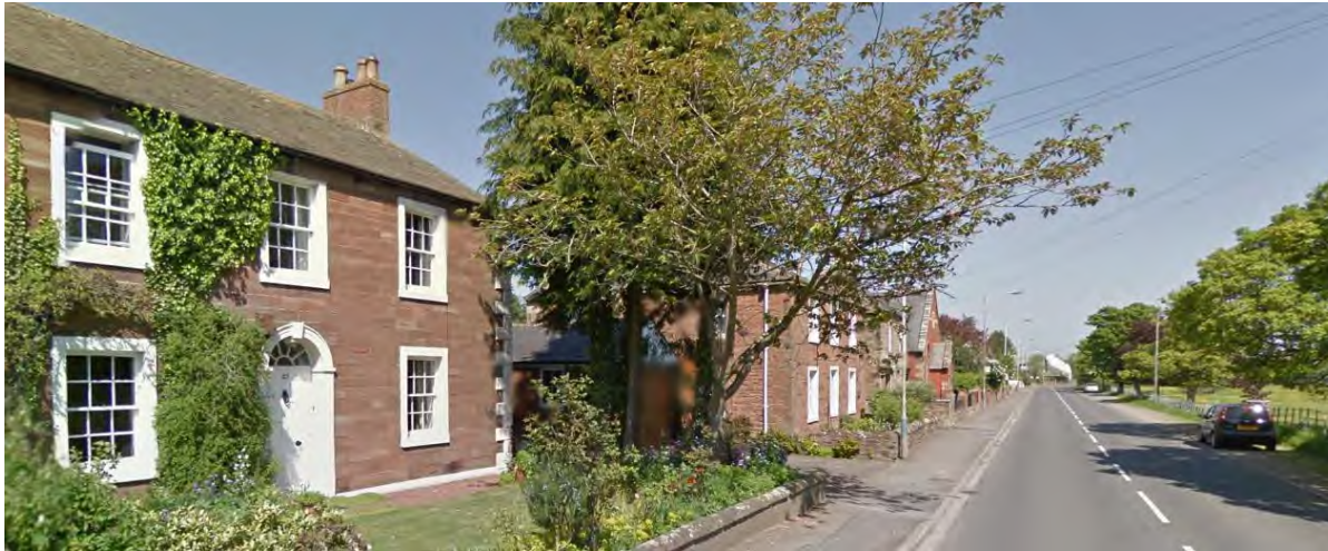
4. Looking north towards The Square. Listed residential properties on The Green, overlooking the flood meadow.
