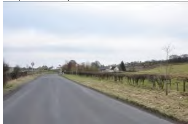
4. View towards settlement from minor road from west showing 30mph gateway. Land falls to river valley, obscuring views of most of the settlement.
