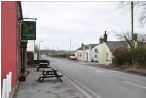
1. Robin Hood Inn at the intersection in the village, where the minor road crosses the A6071. Road edge properties form nucleus of original settlement on long, straight main road.
