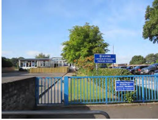
6. Entrance to Scotby School off Park Road.
