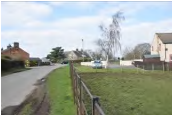
8. Southern end of village viewed from road south east from A595. Gable end of the pub forms the gateway to the village. Smiddy Croft on the right has extended the village further on this side.
