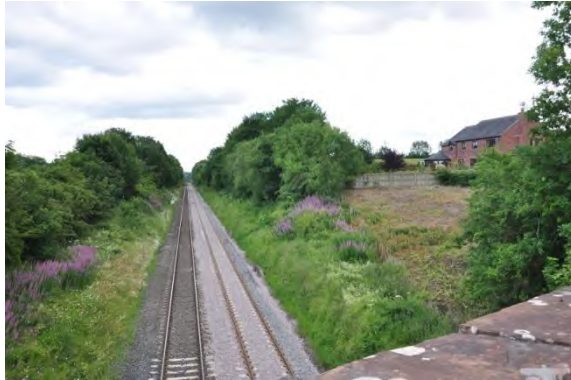
1. The railway cutting is a definite eastern edge to the settlement that extension in that direction is discouraged, although vegetation on the banks is a useful screen for development west of the line.
