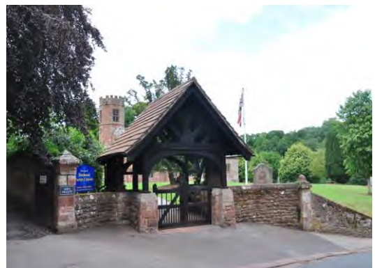
5. Entrance to Holy Trinity and St Constantine central to the historic core of the village.
