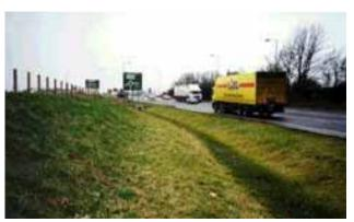
Fig 28. SUDS incorporated into a new highway as an infiltration swale, minimising the burdening of drainage systems.
