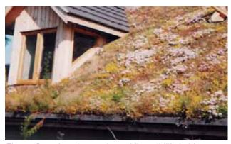
Fig 98 'Green', sedum roof, providing wildlife habitat, slowing rainwater run-off and providing additional insulation.
