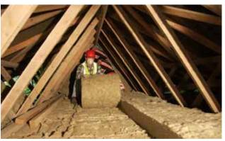
Fig 94. High levels of insulation is one of the key components of a sustainable building. 270mm of insulation is currently recommended. Energy Saving Trust
