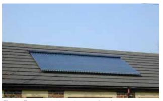
Fig 96. Evacuated tube solar water heating.
