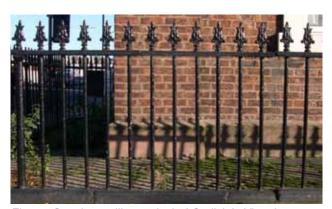
Fig 36. Cast iron railing typical of Carlisle's Victorian terraces. Hawick Street.
