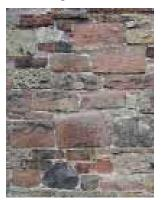
Fig 61 Dressed rubble sandstone walling,
