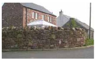
Fig 33. A new random rubble boundary wall in local sandstone appropriate to rural Cumwhitton.
