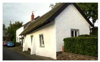
Fig 57. Thatched roof, cob-walled building, Burgh-by-Sands, historically typical of the Solway Plain.
