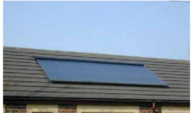
Fig 96. Evacuated tube solar water heating.
