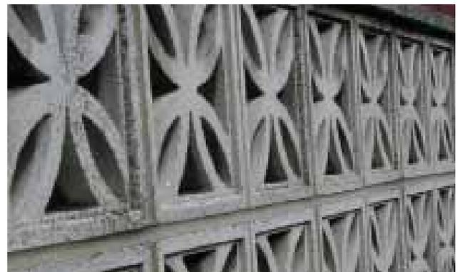
Fig 40. Breezeblock walling is unlikely to make an appropriate boundary treatment in areas visible to public view.
