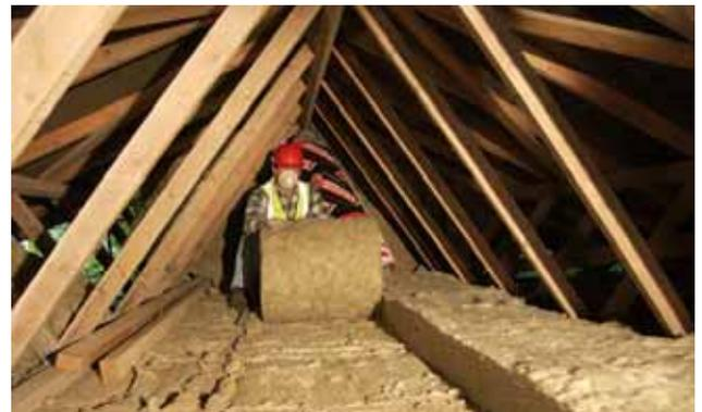
Fig 94. High levels of insulation is one of the key components of a sustainable building. 270mm of insulation is currently recommended. Energy Saving Trust
