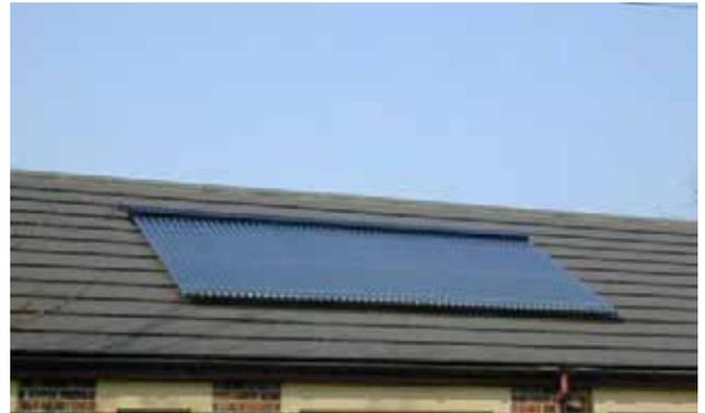
Fig 96. Evacuated tube solar water heating.
