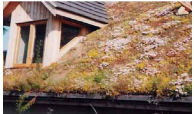
Fig 98 'Green', sedum roof, providing wildlife habitat, slowing rainwater run-off and providing additional insulation.
