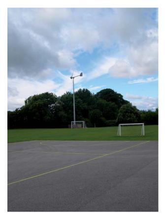
▲ 15 m high, 5kW wind turbine at a south Carlisle primary school powers an air source heat pump for the hall and helps to cut electricity bills
