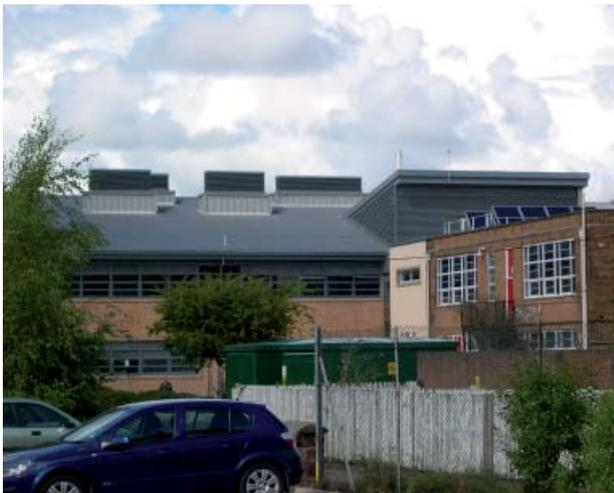
◀ The erection of a technology/science block (2010) at Trinity School, Carlisle provided the opportunity to design in the features of natural ventilation/night cooling stacks, solar collectors and a rainwater harvesting system(below) which gives an instant read out of energy production at the school. ▶
