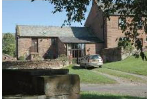
The very simplest provision for vehicular access is appropriate here
