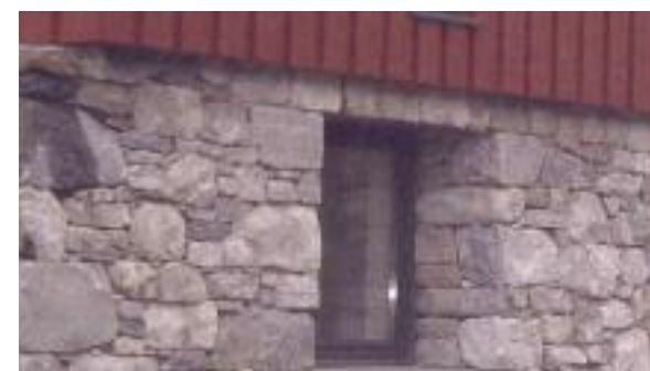
Deeply recessed windows are well protected from wind and rain
