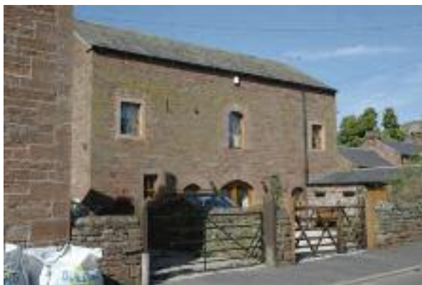
A simple reticent conversion of a Cumbrian barn using existing openings with little loss of character. The retention of boundary walls and gates helps
