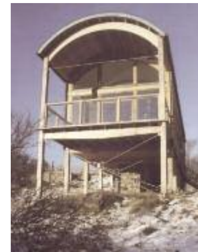
Timber framed home with barn-like roof in profiled sheet and timber cladding
