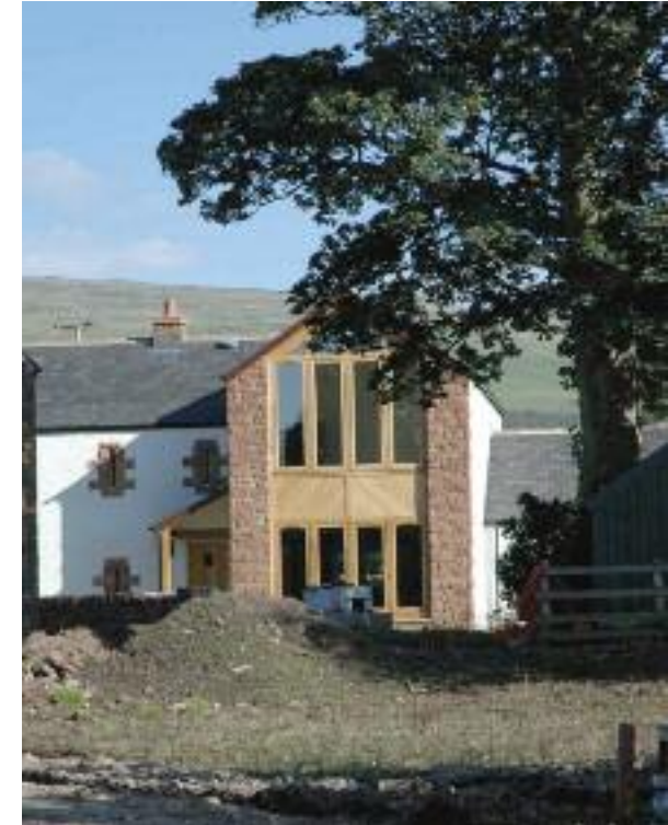
This two storey extension, partly because of its position and manner, has come to dominate the original house behind
