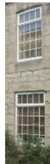
These uPVC windows are not traditional in style with their top-hung opening lights and their stuck-on glazing beads. They are also set too far forward in the window reveal
