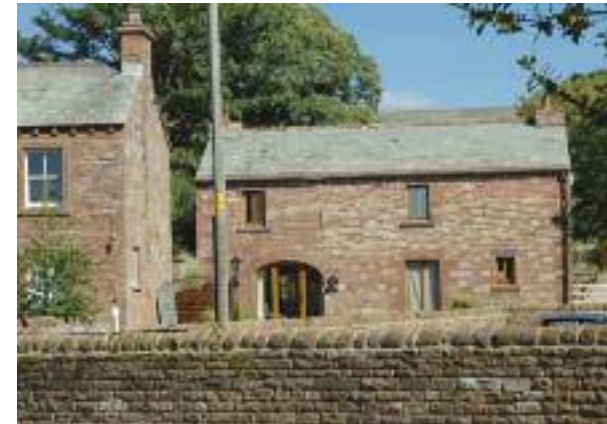
Westmorland slate roof often graded in diminishing courses
