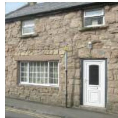
This uPVC door tries to emulate traditional detailing and style but fails miserably. Two different styles of window have been used, the lower one far too wide and with inappropriate ‘stick-on’ glazing beads
