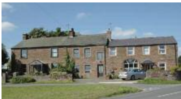
The conversion of the barn on the right of this group has destroyed its character with fussy porch and intrusive windows
