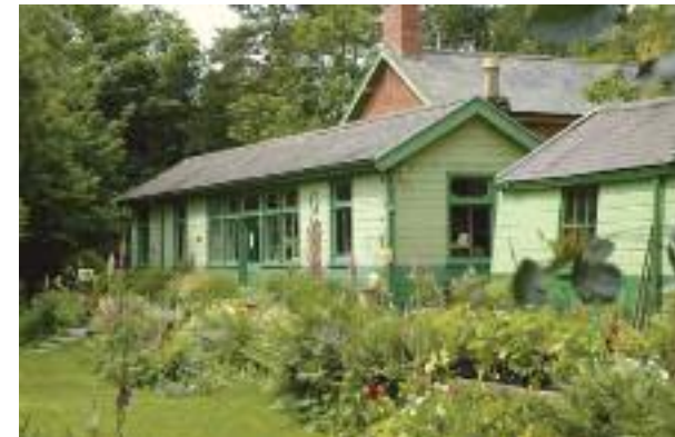
Welsh slate on this attractive group of Edwardian buildings at Garden Station, Langley
