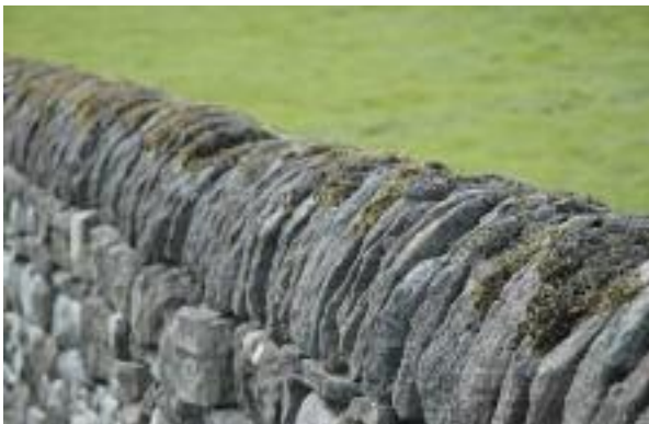
Neat roughly rounded capping stone to this dry stone field wall
