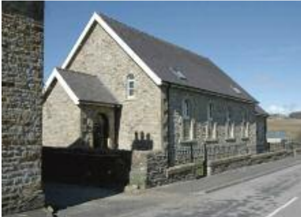
A robust stone porch with a slate roof matching the main roof material and pitch
