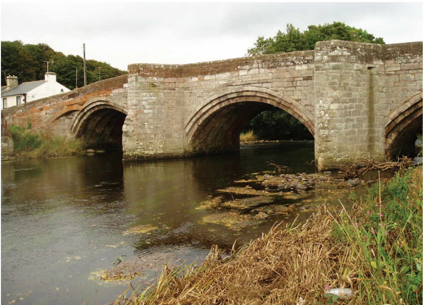
↑ Eamont Bridge (above and left)
