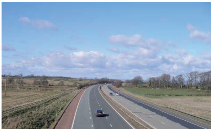
▲ The M6 motoway, south of Junction 42.
