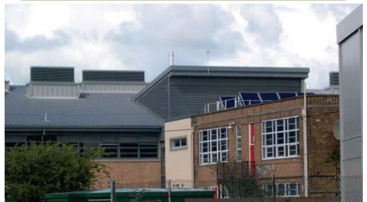
Trinity School Solar Panels ►
