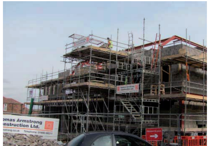
▲ Sainsbury's, Scotland Road, under construction.
