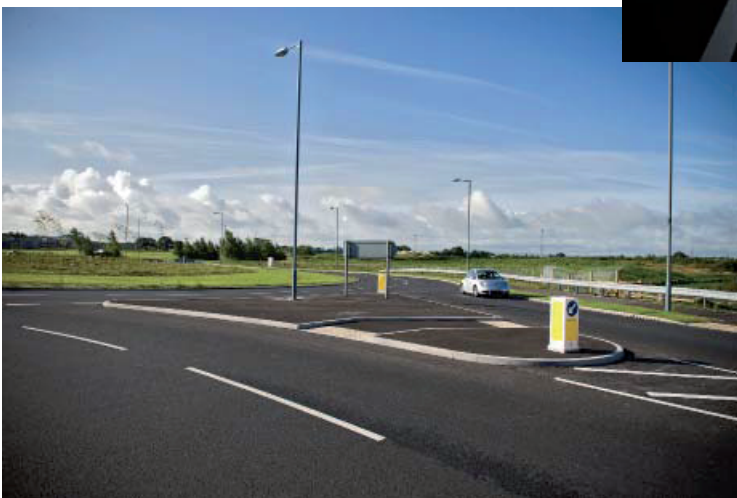
▲ Carlisle Northern Development Route © Cumbria County Council
