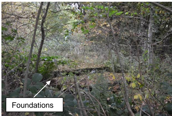
Plate A.6: Building foundations within woodland
