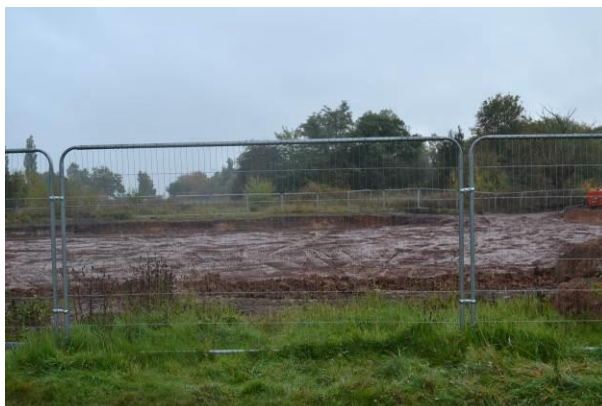
Plate A.10: Construction site
