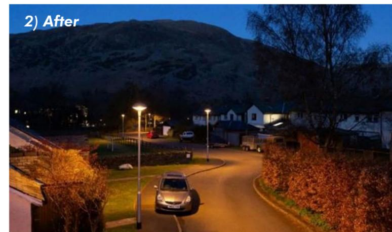
**Glenridding** lighting project used Night-Tune luminaires specially developed to utilise adaptable warm colour temperature at lower mounting height whilst allowing safe access & legibility throughout the site.
