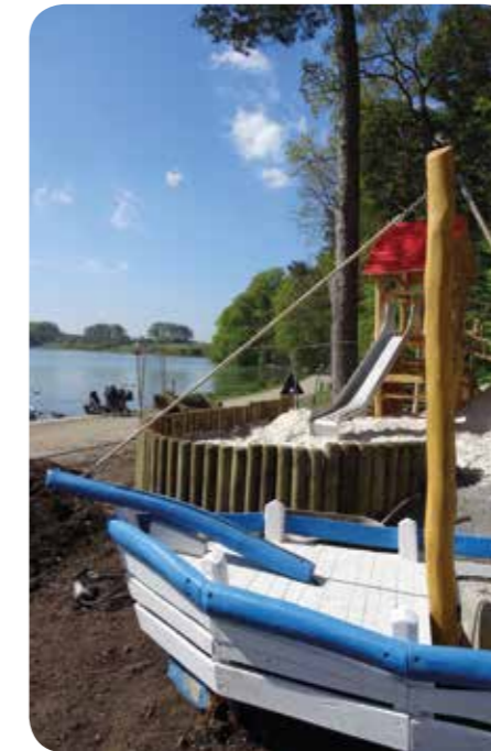
Above: Work underway on the Talkin Tarn play area
