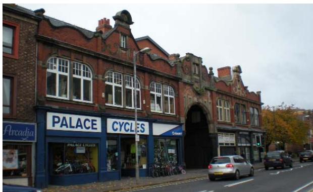
Fig 33. The Palace Arcade building - sadly missing a pediment previously located over the central arch.
