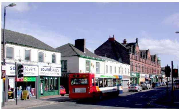
Fig 02. Botchergate has a legacy of both grand and modest commercial buildings, but with many marred by poor quality alterations.
