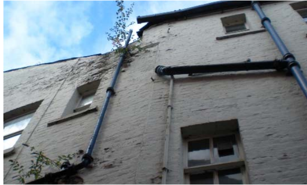
Fig 44. neglected maintenance of gutters leading to vegetation growth and likely damage to building fabric.
