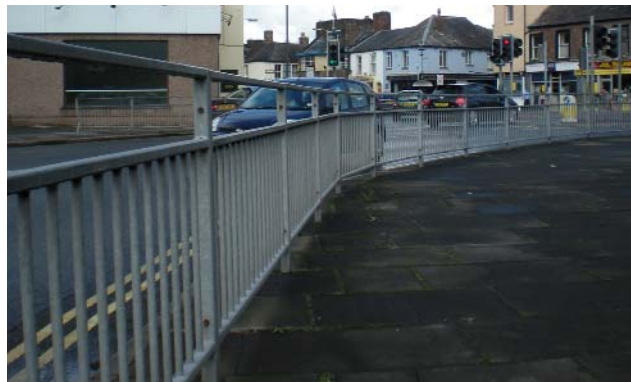
Fig 55. Guardrailing at St Nicholas Street.
