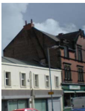
Fig 30. Truncated chimney stack to the Stanley Hall.
