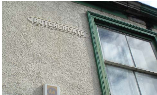
Fig 56. A cast iron street nameplate which could readily be restored, adding some quality to the streetscape.
