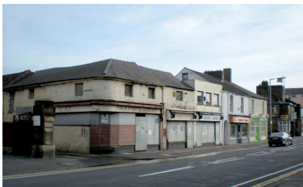
Fig 29. An unimplemented permission exists for this block between Rydal and South Henry Street.
