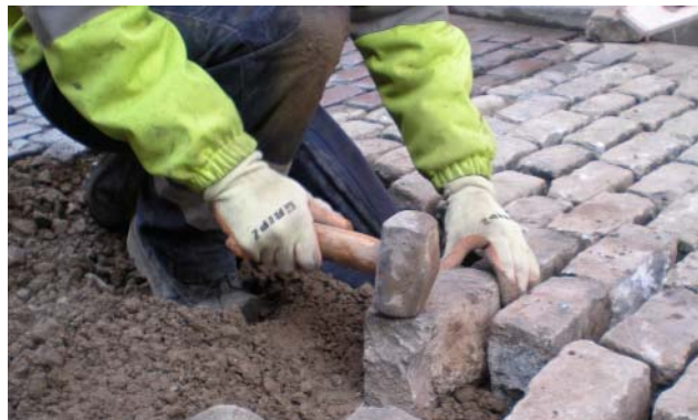
Fig 57 Restoration of Setts on Collier Lane.
