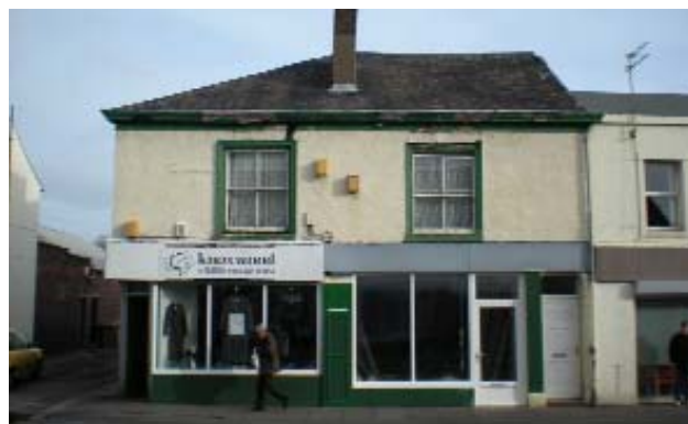
Fig 60. 107-109 Botchergate which although having lost their original shopfronts, retain original sash windows capable of refurbishment.
