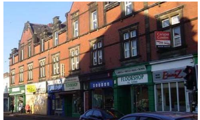
Fig 08. The 1905 Stanley Hall - a prominent Edwardian building in 'Area 2' (prior to refurbishment)
