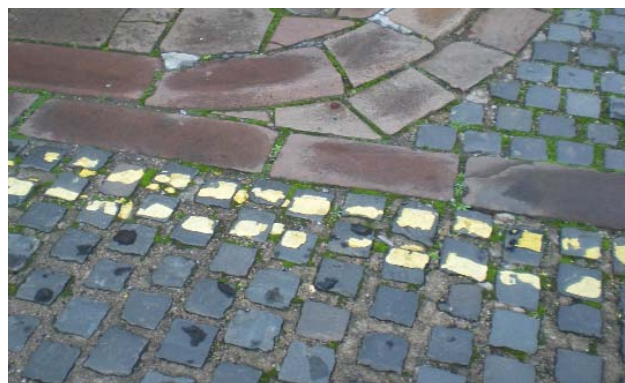
Fig 40. Setts and sandstone kerbs and paving at Mary Street.
