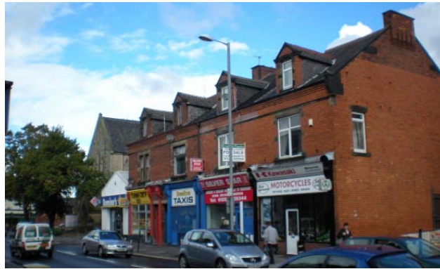
Fig 36. More sympathetic signage and reinstatement of appropriate window designs would lift this row considerably.
