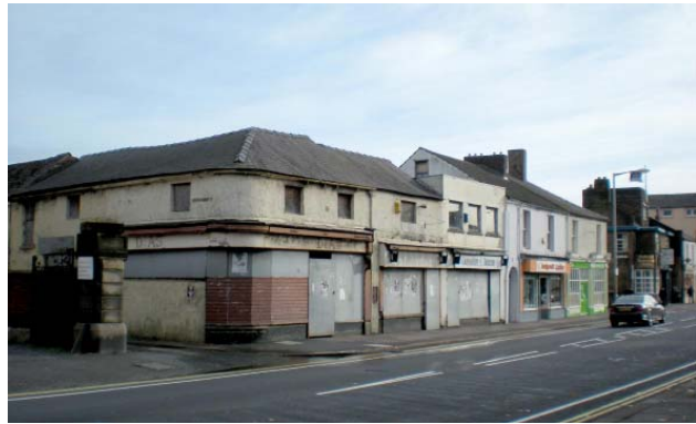
Fig 29. An unimplemented permission exists for this block between Rydal and South Henry Street.
