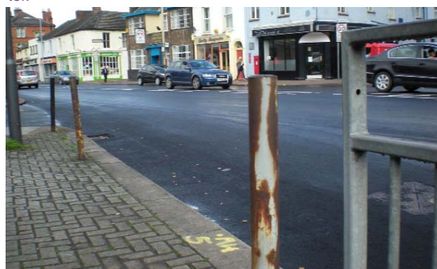
Fig 42. Unsightly bollards and guardrailing close to St Nicholas Street.
