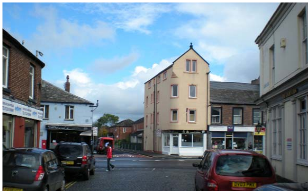
Fig 19. A prominent building at 1 London Road, which has recently has render applied over its original brickwork
