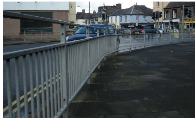
Fig 55. Guardrailing at St Nicholas Street.
