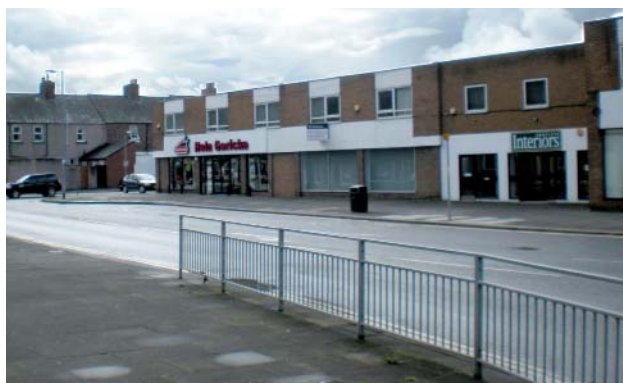
Fig 64. 12-18 St Nicholas Street - although outside the current conservation area is a site whose enhancement would be of great benefit to the wider area.
