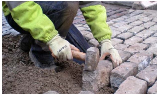
Fig 57 Restoration of Setts on Collier Lane.
