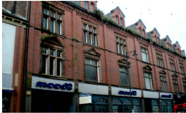
Fig. 61 The large vacant 'Mood' building could be subdivided to provide smaller retail units with upper floors suitable for residential or office space. effectively behind the retained facade of the fire-damaged building.
