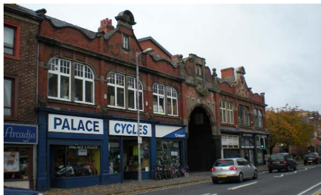
Fig 33. The Palace Arcade building - sadly missing a pediment previously located over the central arch.
