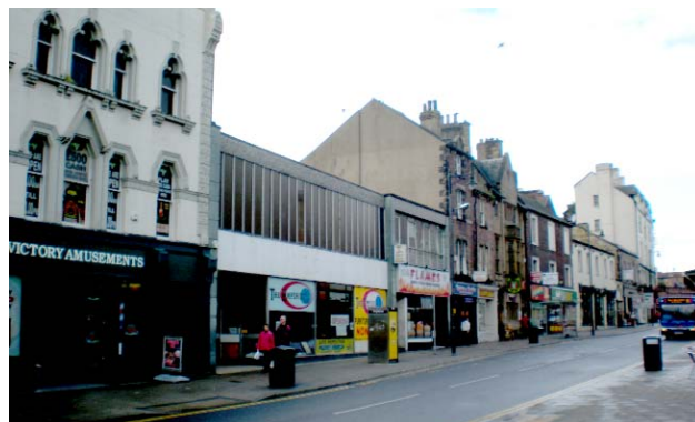
Fig 03. An incongruous 1960s structure, with significant potential for redevelopment.
